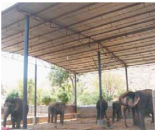
Figure 3a: Better shade, with the enclosure roof being 25 feet high.
