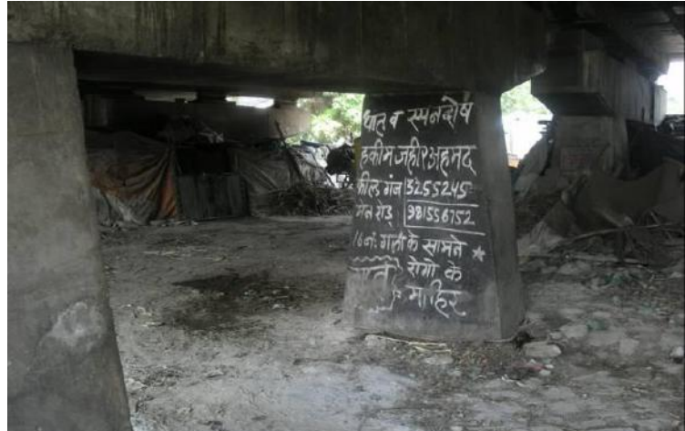
Figure 3: Unnatural and unhygienic flooring.
